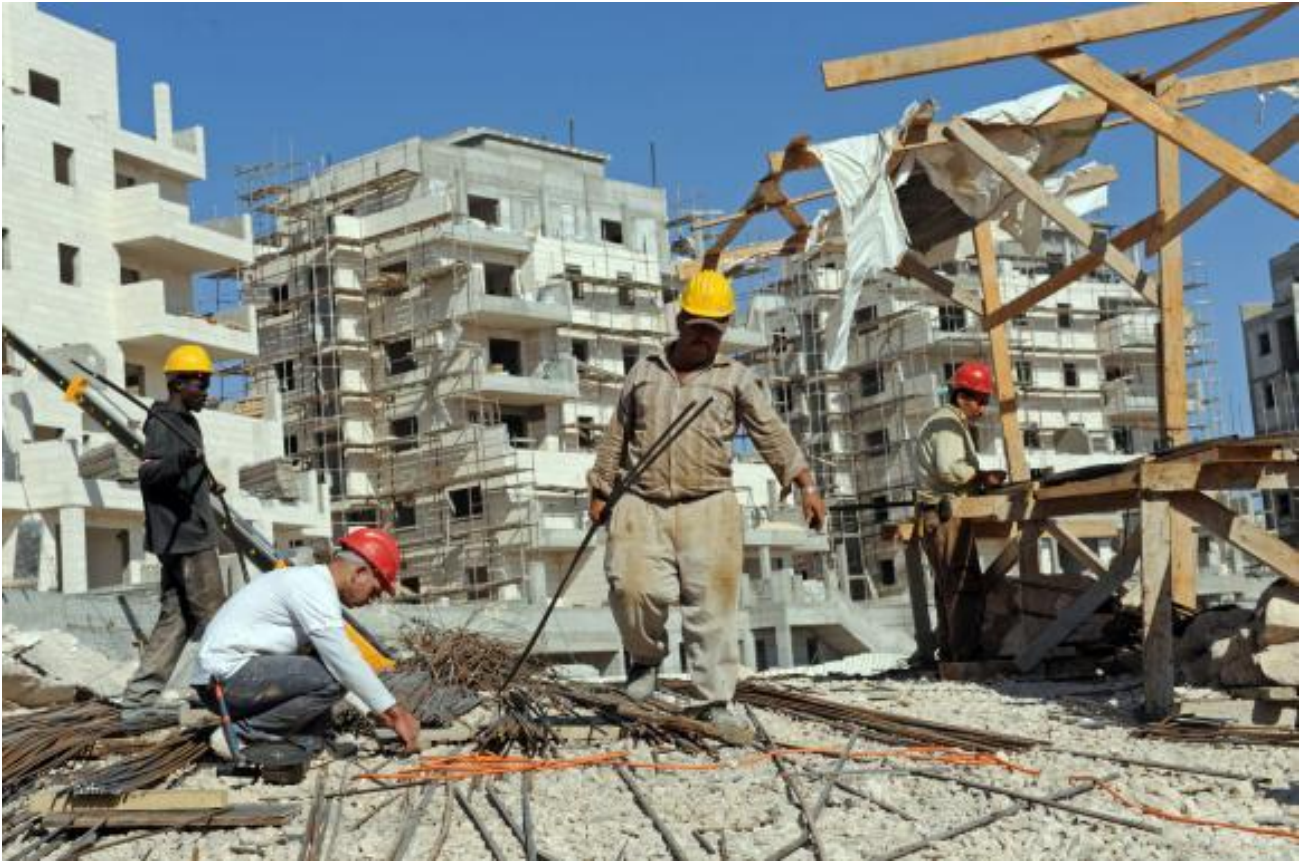
Figure 7. Palestinians at work building the illegal Israeli settlement of Har Homa that separates East Jerusalem from Bethlehem. Unfortunately due to the Israeli occupation these are frequently the only jobs these workers can find; to add insult to injury they are denied union representation despite being made to pay an organising fee to the Histadrut.
